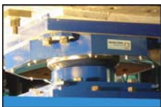
Fig. 5: Example of an isolation device manufactured by Maurer Söhne, Germany. This device allows relative displacements between the foundation and the structure.
