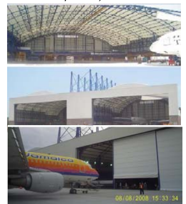
Fig. 4 Top: Hangar roof structure, formed by light-weight steel frames, and semitransparent roof cover providing abundant natural light. (span: 44 m). Center: Hangar front view. Below: Vertical sliding doors are being opened.
